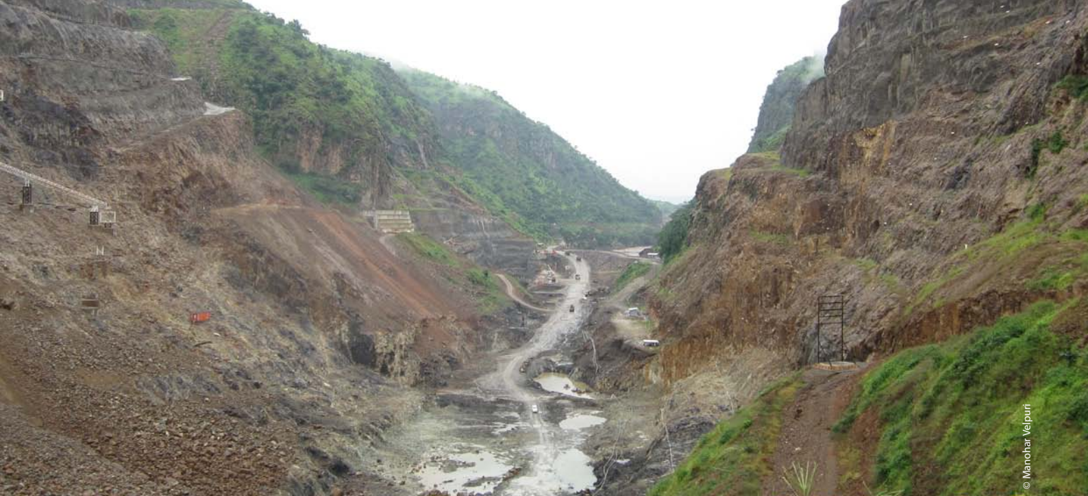
Gibe III dam site (as of April, 2011).
