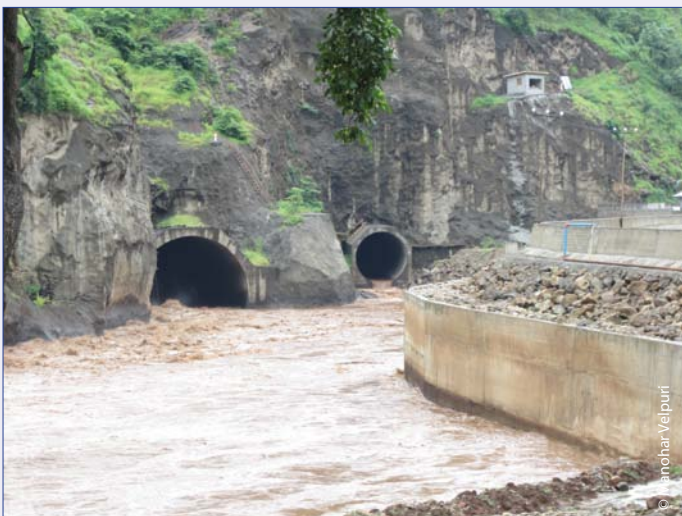
Diversion tunnel outlet.
