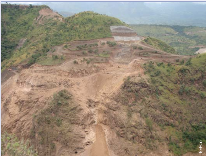
Left bank dam excavation.
