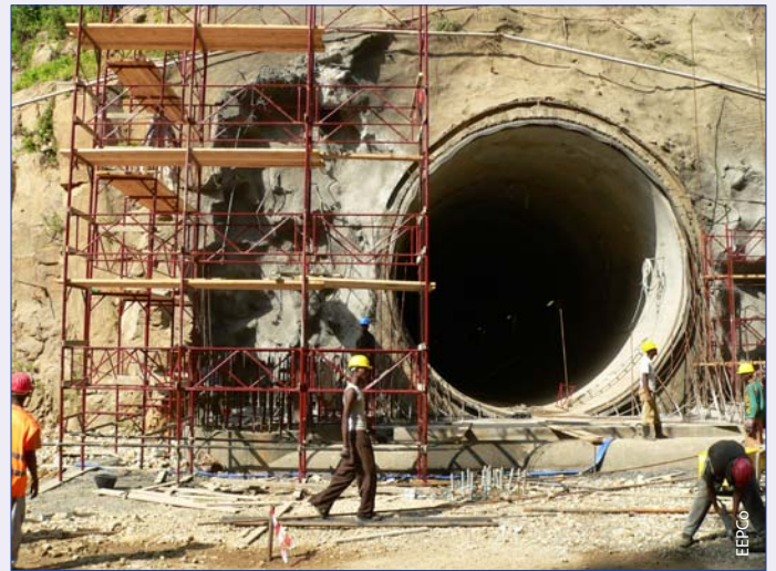
Work on a diversion tunnel.
