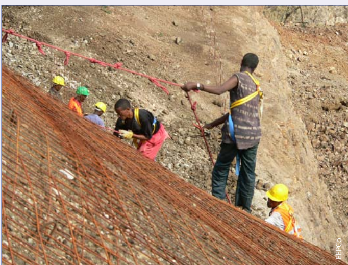
Workers on the dam abutment excavation.
