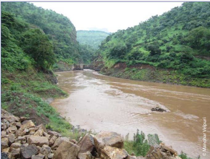
Diversion tunnel inlet canal.
