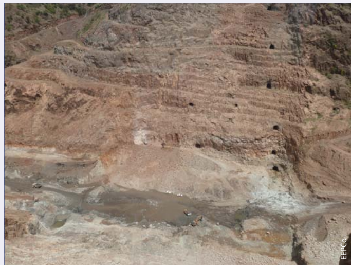
Looking down into the construction site (right abutment dam excavation).
