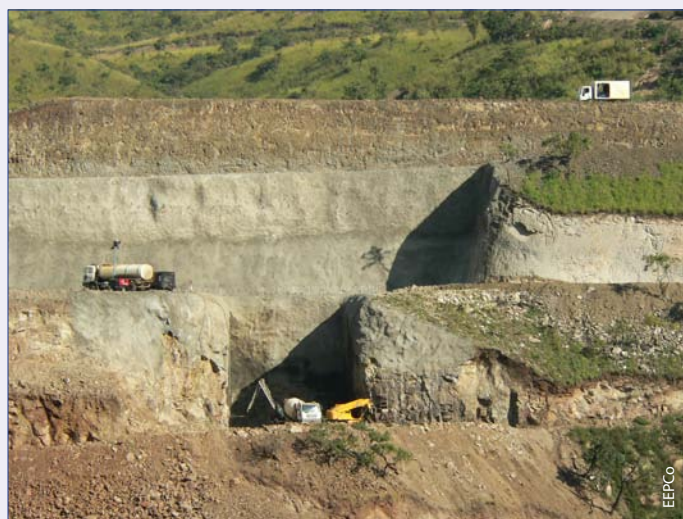
Left bank dam excavation.
