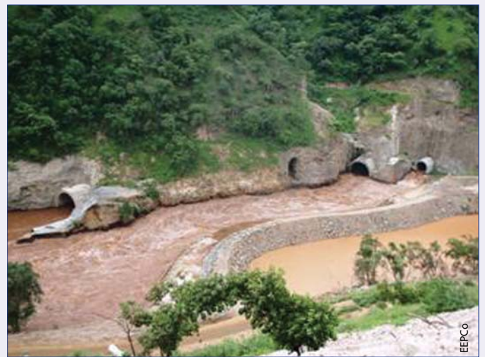
Diversion tunnel outlet.
