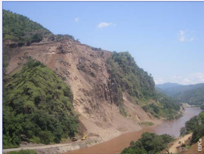
Roads along the Omo River leading to construction site.
