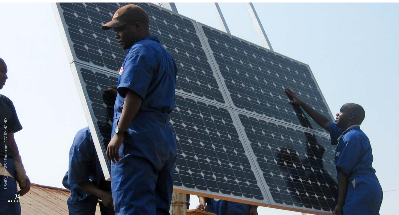
Workers installing solar panels
