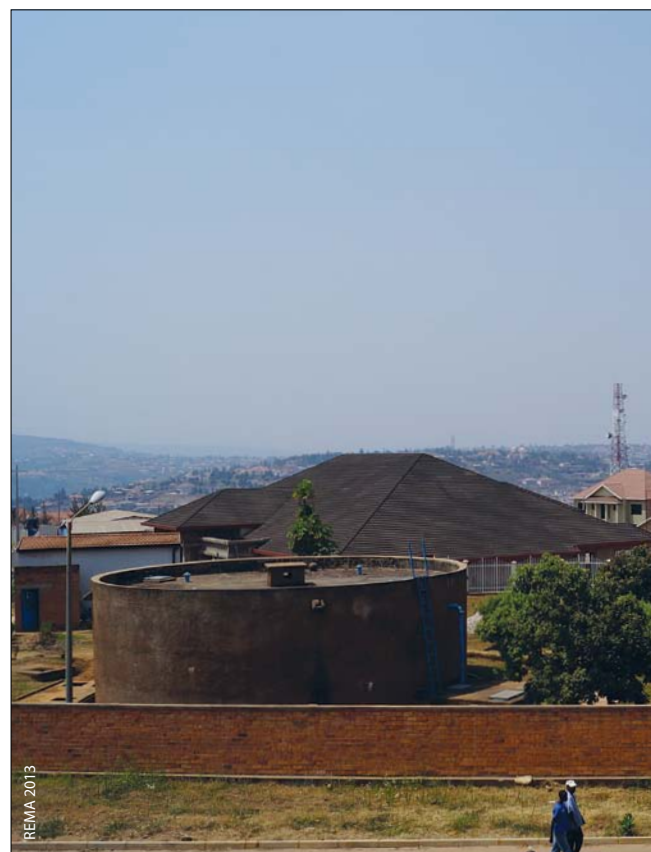
Water storage tanks supplying the Gacuriro neighbourhood
