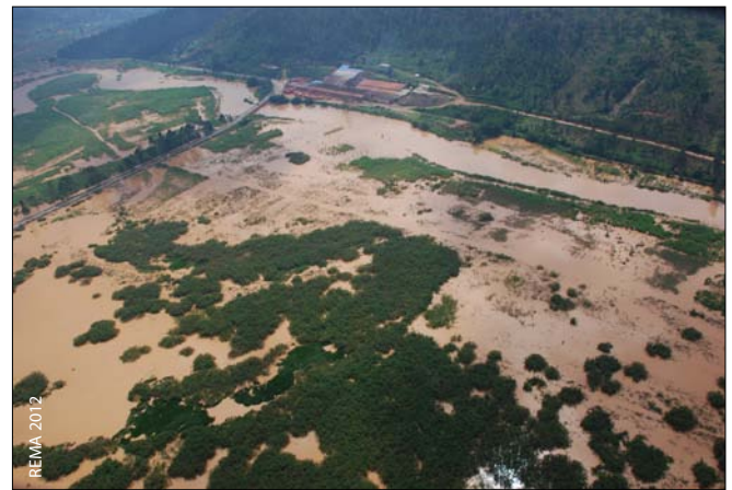
Flooding at Ruliba Clays
