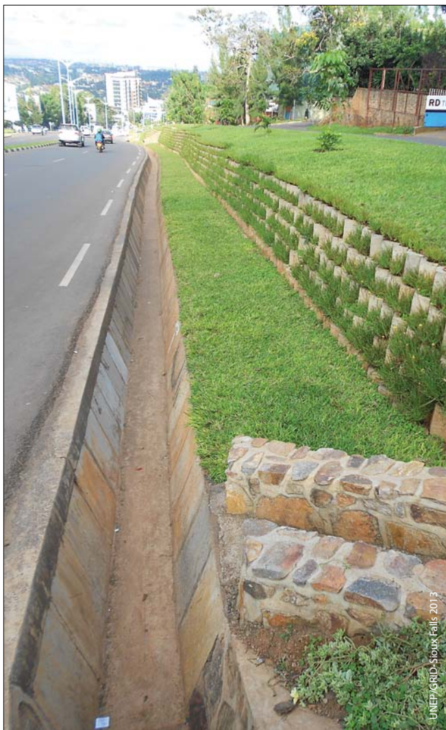
Green, grassy retaining wall along one of Kigali's busy streets
