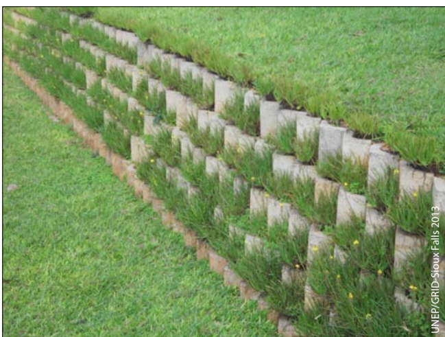
Terraced green walls, such as the above, help to absorb rainwater and prevent soil erosion along streets
