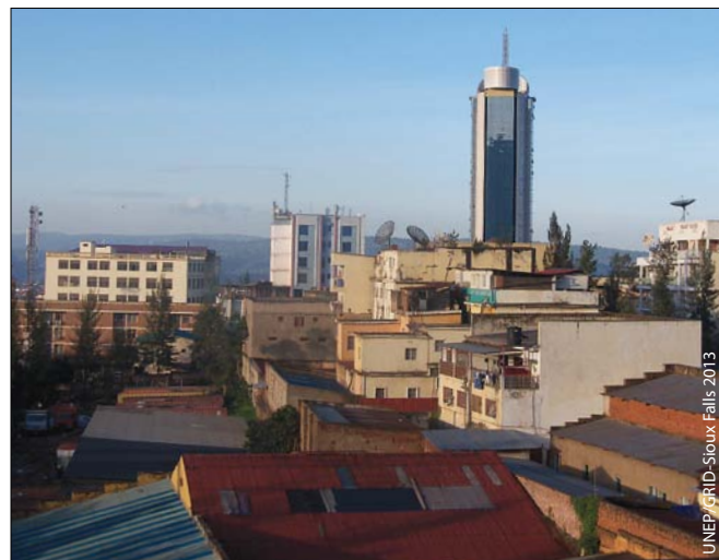
Kigali City Tower, located in Nyarugenge Sector, surrounded by the old commercial and mixed-use buildings, most of which have already been vacated for demolition to make way for new designated land uses according to the KCMP
