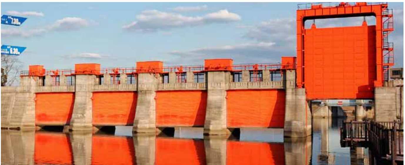
The historic Iwabuchi floodgate, in Tokyo, remains crucial for communities living along two of Japan's rapidly-flowing, flood-prone rivers. © Juergen Sack
