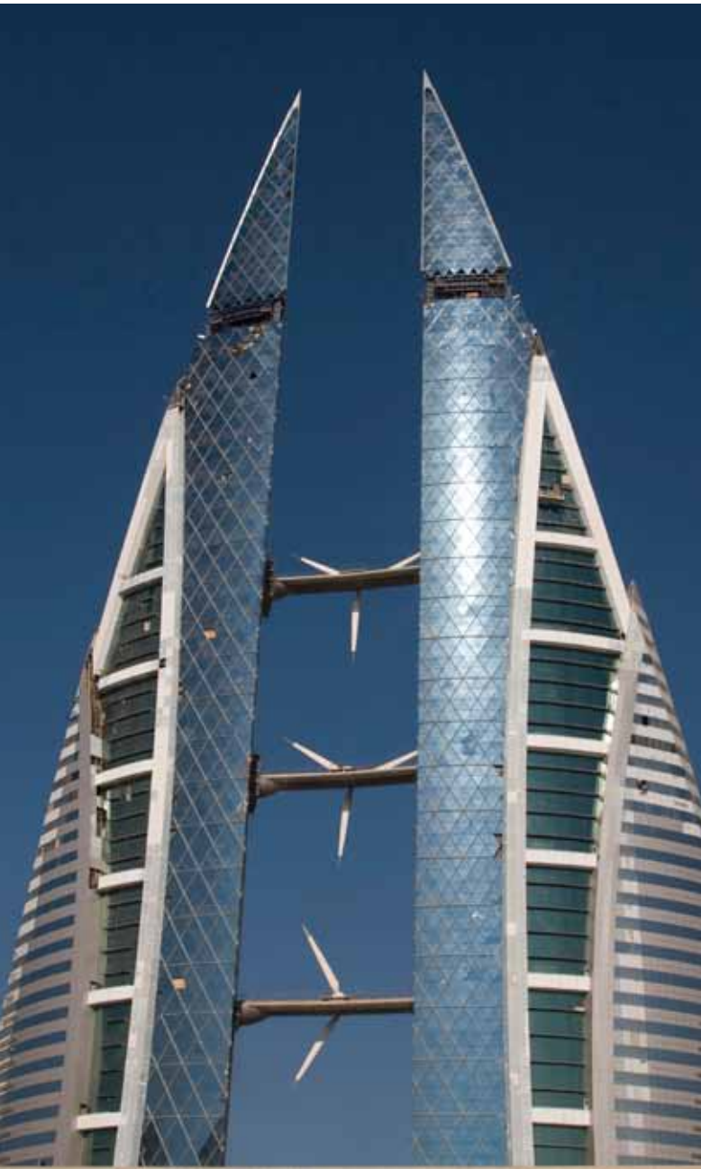
Featuring three integrated wind turbines, the Bahrain World Trade Center boasts the world's most sophisticated skyscraper energy recovery system. © Klaas Lingbeek- van Kranen
