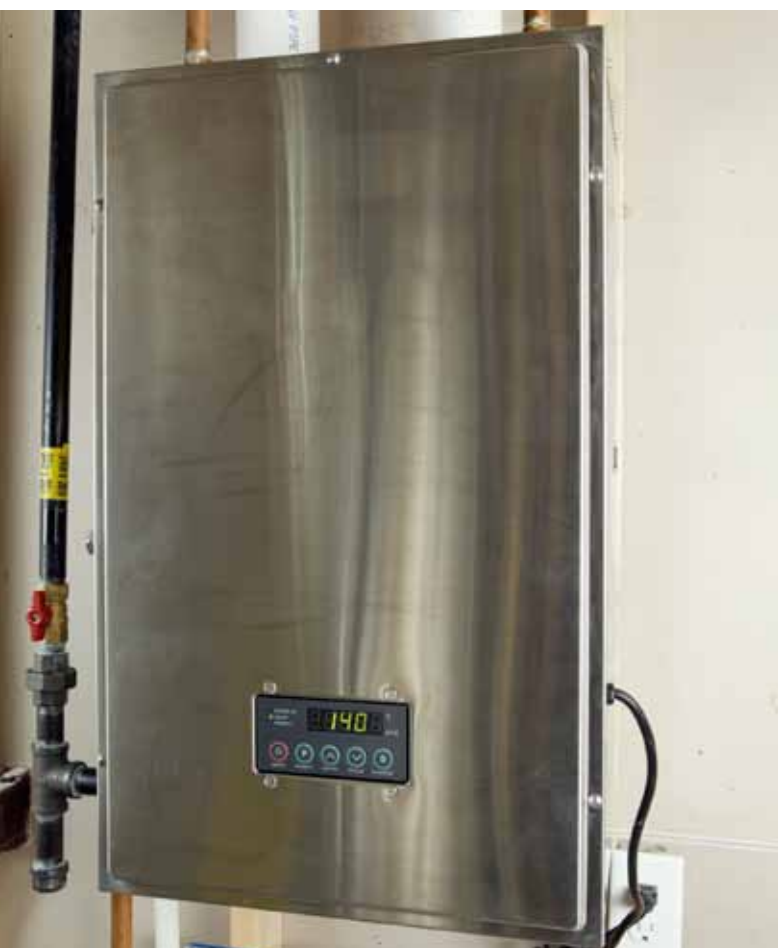
A residential condensing hybrid tankless water heater. This technology produces hot water on demand and is much more energy efficient than a conventional hot water holding tank. © BanksPhotos/iStock
