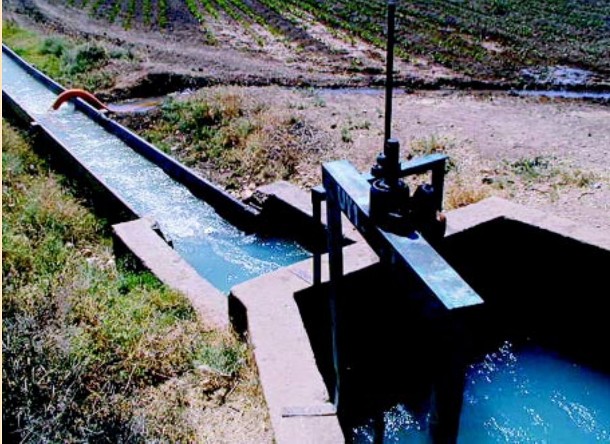
A siphon off-take irrigating a field in the Harran Plain. Photo courtesy of the United States Foreign Agriculture Service.
