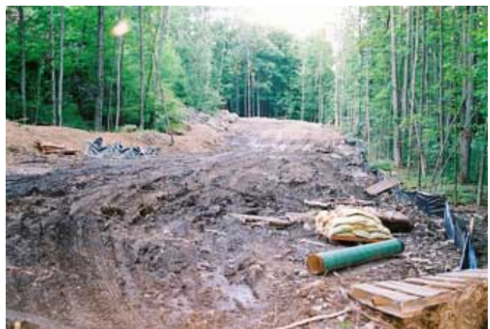
Drilling requires the clearing of land which alters the landscape. Here, trees have been cleared to build a road to reach the drilling site.
