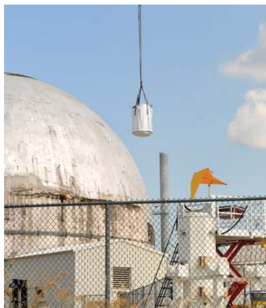
Removal of nuclear waste from a reactor of a military research programme site. (Photo by Argonne National Laboratory www.flickr.com )
