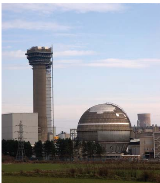
Dismantling of the tower of a military reactor. (Photo by Tim Duckett www.flickr.com )
