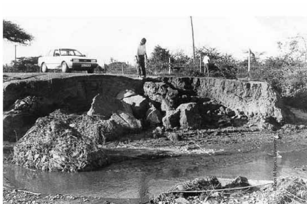
A section of Massii-Makueni highway where a major bridge was destroyed in a late 1990s land slide
